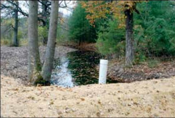
*The check dam is a small dam with an overflow pipe connected to a culvert beneath the dam. These check dams will slow down the flow of the water and allow sediment to collect in the basin of the check dam versus flowing directly to the lake. Sediment like this has phosphorus attached to it, the nutrient that fuels algae blooms in the lake.*
