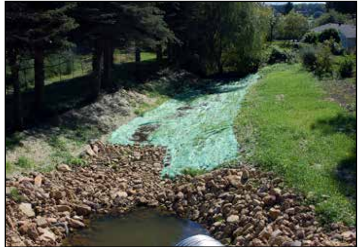
Left: Overgrown and eroding stream on the Pullen property. Above: After installation of a design to reduce phosphorus in runoff from entering the lake.
